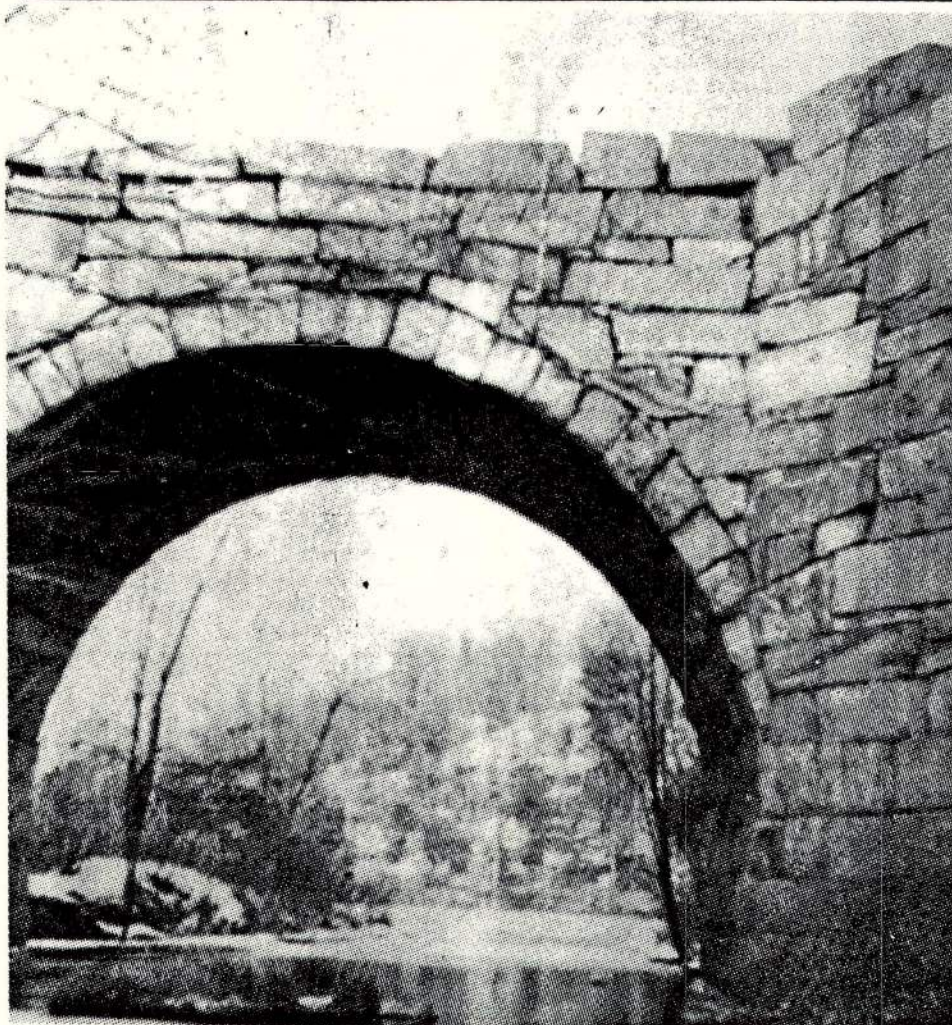
The Stone Arch Bridge, built around 1872 as part of the Nashua, Acton, and Boston Railroad, extends across Stony Brook halfway between Forge Village and Graniteville. It is made of local granite; no mortar was used in construction. (Photo from Sept. publication of WESTFORD RECOLLECTIONS 1729-1979.) (A Gagnon photo from the WESTFORD RECOLLECTIONS Series.)
