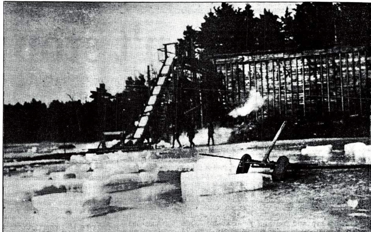
The thickly frozen surface of Forge Pond creates a fertile harvest for ice workers at the turn of the century. Wooden rollers form a conveyor belt for the blocks of ice, lifting them into the storage facility at the site of what today is the town beach.
