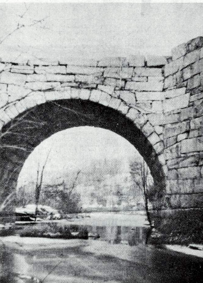
The Stone Arch Bridge, built around 1872 as part of the Nashua, Acton and Boston Railroad, is made of local granite; no mortar was used in construction. (A Gagnon photo from the WESTFORD RECOLLECTIONS SERIES)
