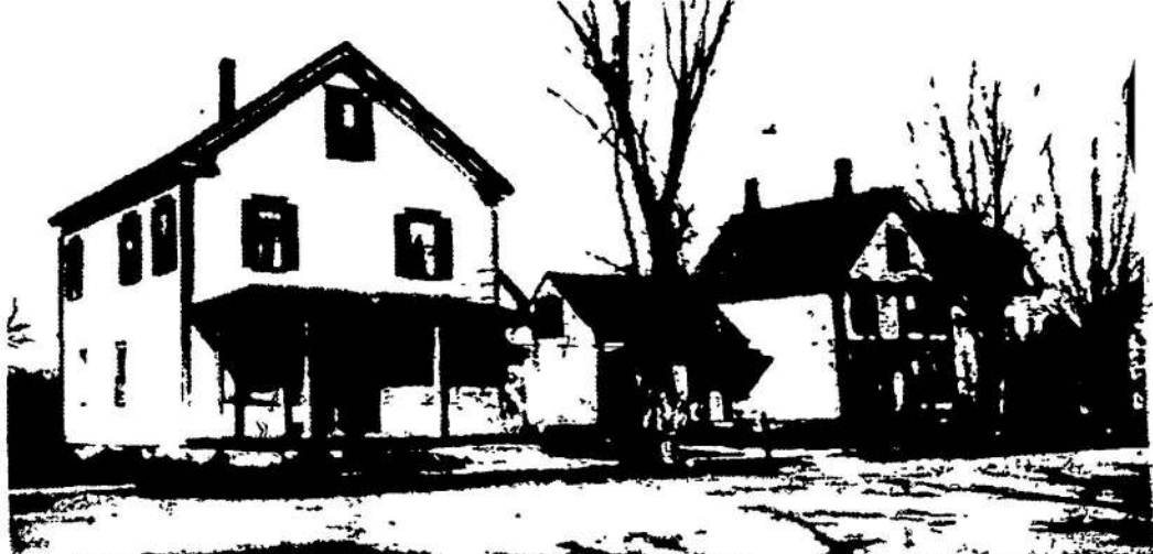
This set of buildings on Main Street, which faced the present Central Fire Station, was the shipping point for Westford fruit going to the Boston Market. The house on the right and a large barn in the rear were destroyed by the fire. The stock standing at the lot adjacent to the Fletcher Library, was demolished in 1944. Photo courtesy of Gordon B. Seavey.
